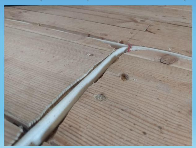
Yes, the cable is less than 1-1/4" from the surface and requires protection. NEC 334.15 (B) Protection from Physical Damage. Cable shall be protected from physical damage where necessary by rigid metal conduit, intermediate metal conduit, electrical metallic tubing, Schedule 80 PVC conduit, Type RTRC marked with the suffix - XW, or other approved means. And also.....
