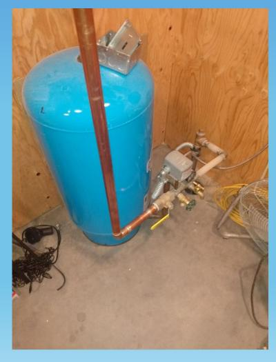
No, this is metal water piping even though it is being used for heat so 250.104(A) is the section to use for bonding of metal water piping not 250.104(B) other metal piping.
